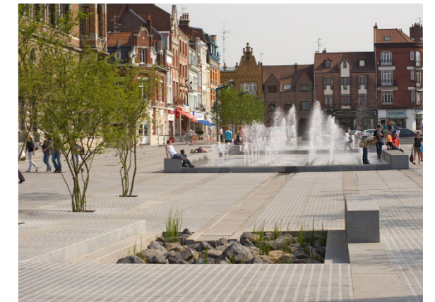
Hard surfaces channelling water to soakaways
