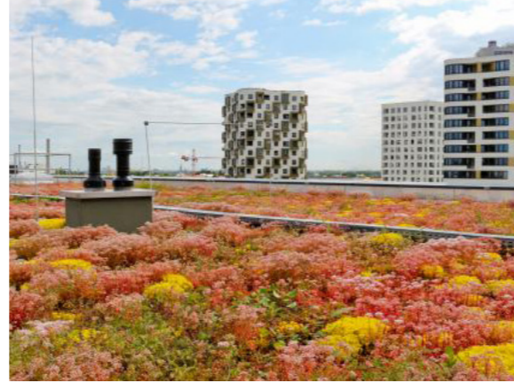
Sedum on the more visible, lower roofs More dependable for year-round appearance
