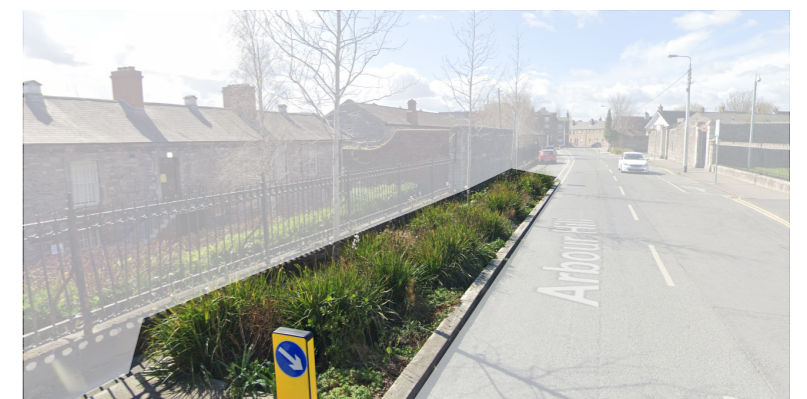
Planting Build-out into carriage way by DCC Parks
